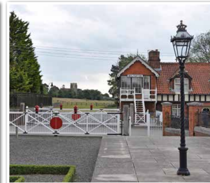
The last Royal Trains ran to Wolferton station in 1966, and when Her Majesty The Queen travels by rail from London to Sandringham House every Christmas, she now goes the last few miles from King's Lynn by car. The ornate station is still maintained in immaculate condition, and the private owner of the eastern platform building welcomes summer visitors. HOWARD JOHNSTON.
